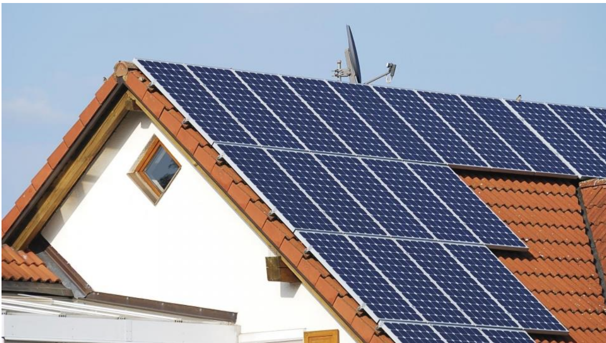
Figure 2 - Photovoltaic power plant on the roof 2
